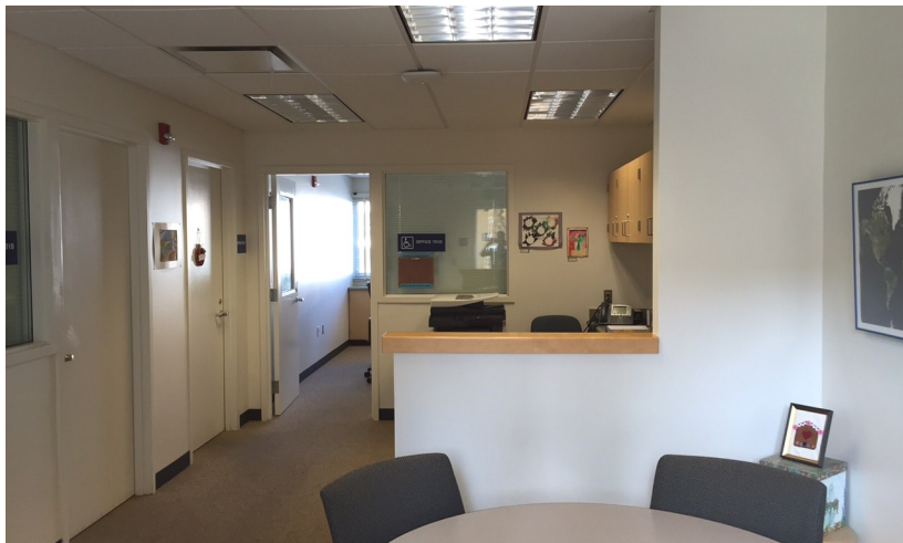
Remodeled support offices
