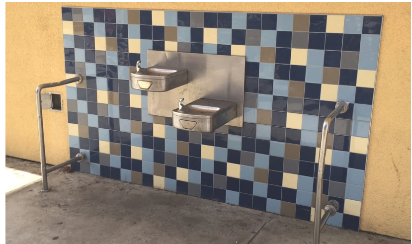
ADA compliant drinking fountain
