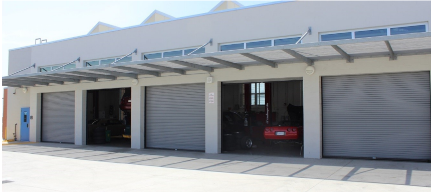
Roll-up doors and bays
