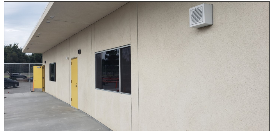
New Relocatable Classroom
