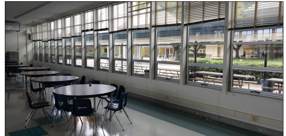
Dining Room - New Window & Light Replacement
