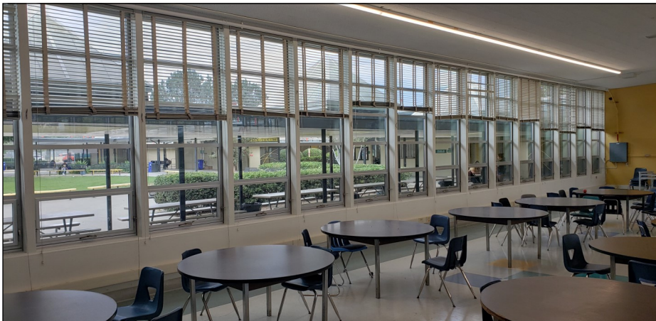
Dining Room - New Window & Light Replacement
