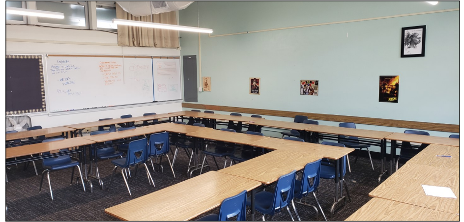
Existing Classrooms - New Carpet & Paint
