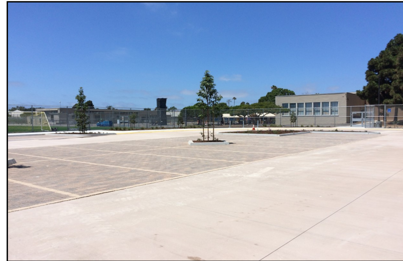
New Parking Lot
