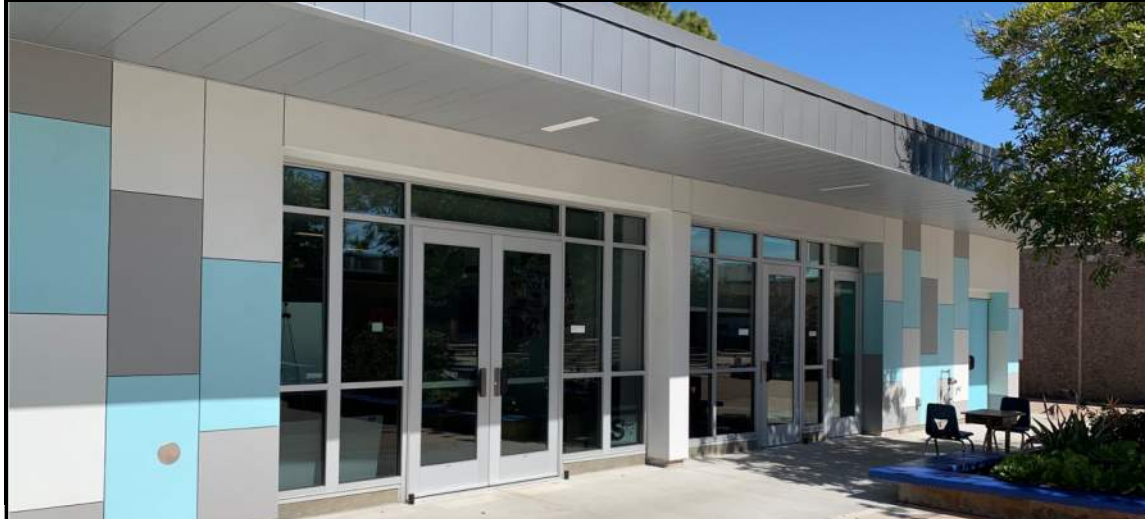
CAMPUS ENTRANCE COMPLETED
