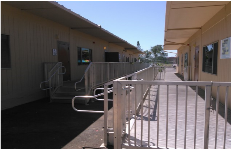
Portable Campus Classrooms
