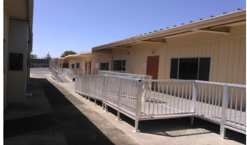
Portable Campus Classrooms
