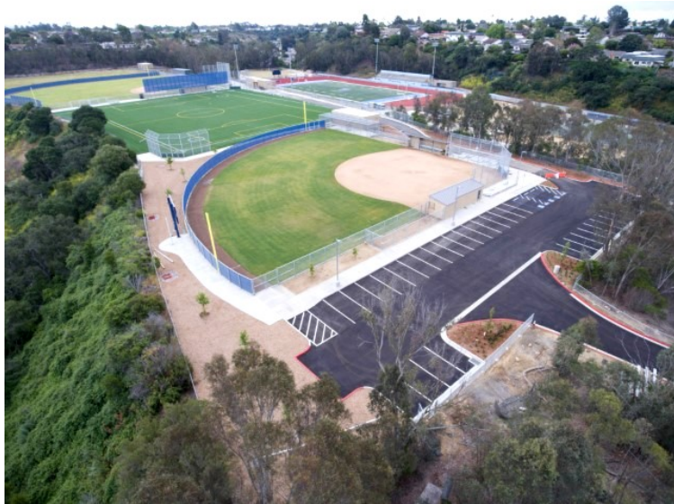
Aerial of upper field with completed upgrades
