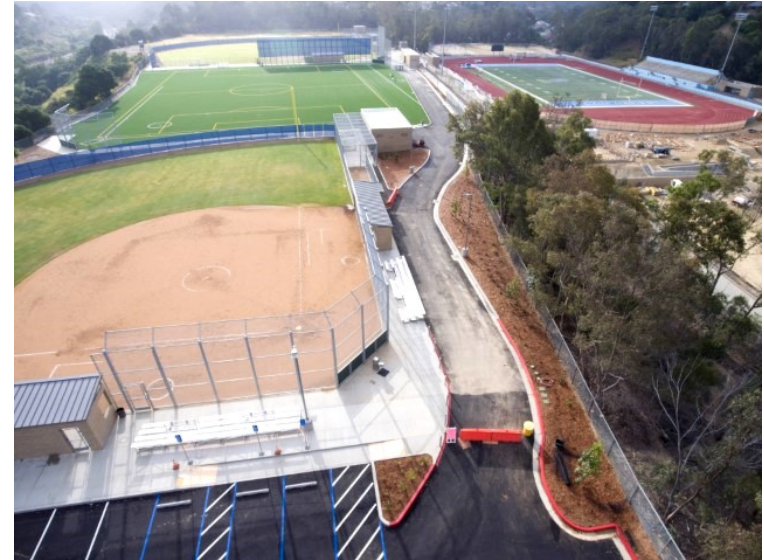
Aerial of upgraded softball field and access road
