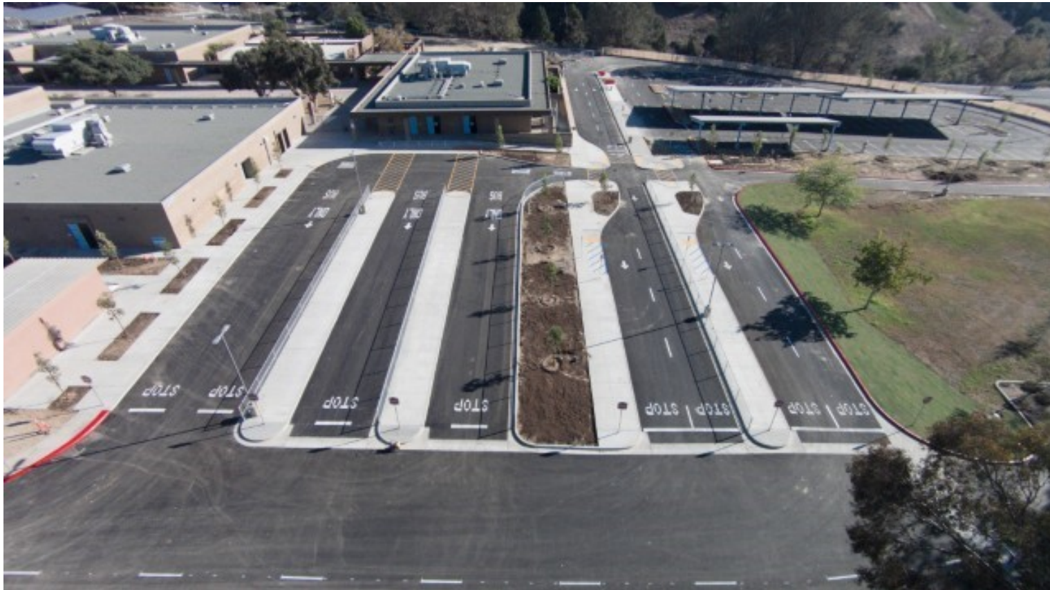
Student/Bus Drop-off Area and staff parking lot is complete
