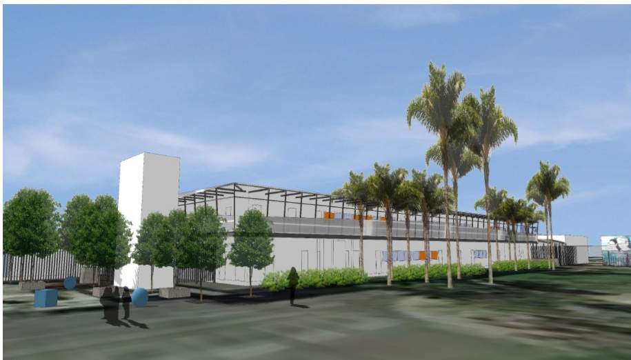
Two-story classroom building view from playground
