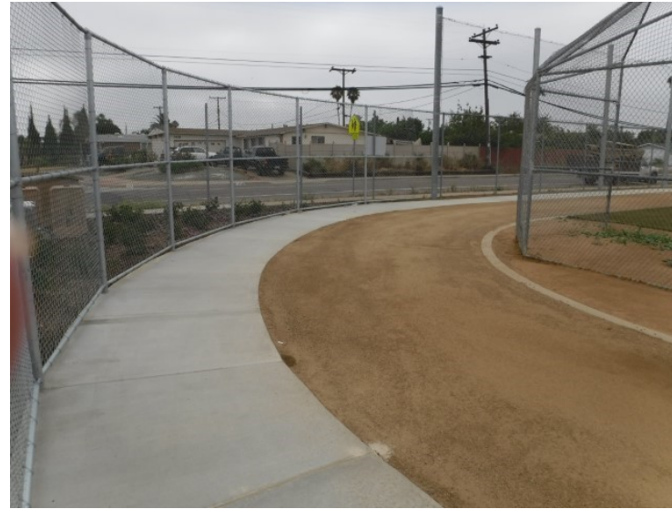
Walkways and Track around perimeter
