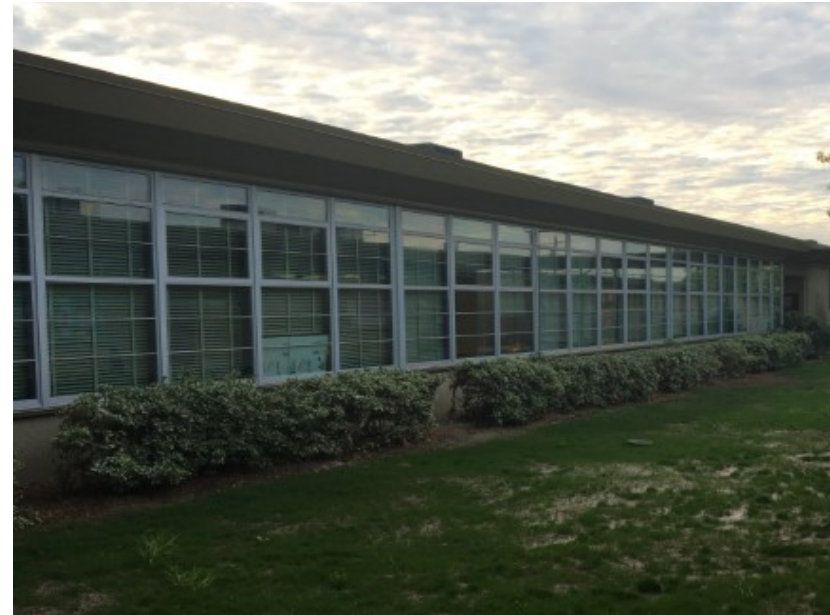
Example of new windows
