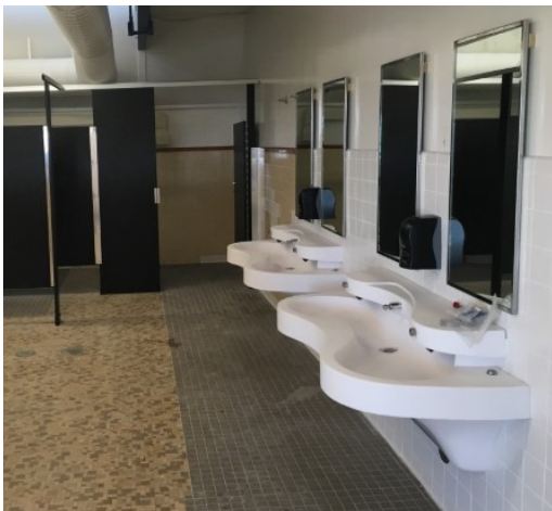
New bathroom fixtures
