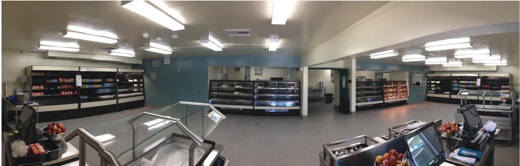
700 building — Remodeled food service area with cold and warm cases and point of sale equipment
