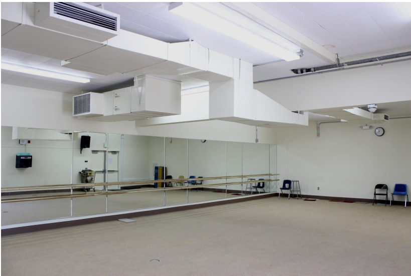
800 building — New PE activity room
