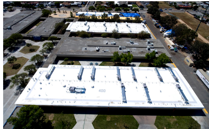
Aerial of work in progress on Phase I
