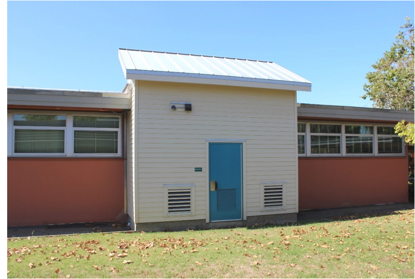
Air conditioning mechanical housing
