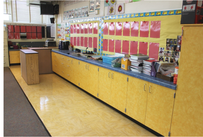
Newly installed classroom cabinetry
