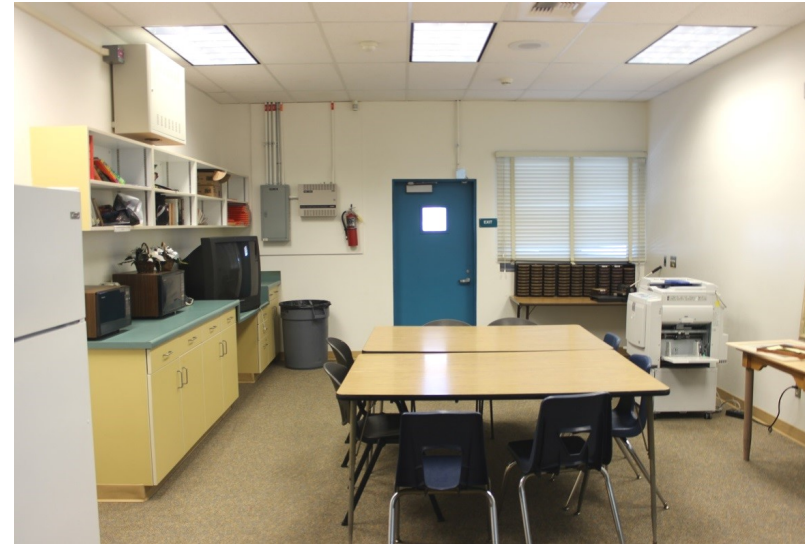
Renovated teachers lounge/break room
