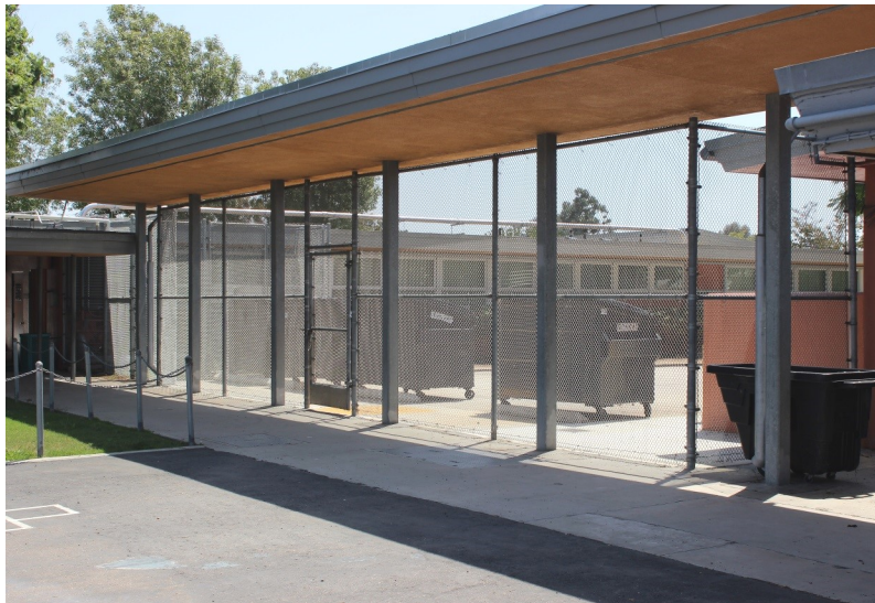
Security fencing upgrades near dumpster area
