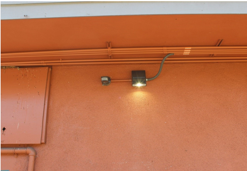
Security lighting upgrades
