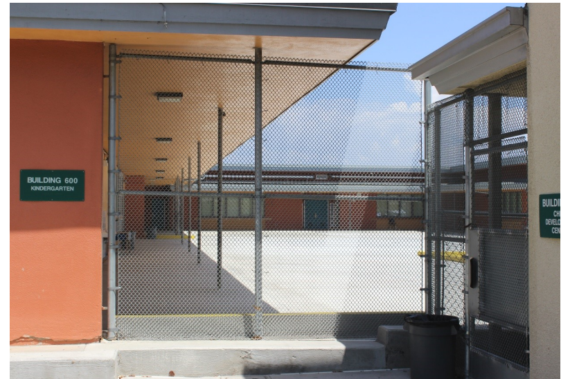
Non-climbable fencing between buildings
