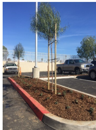
Upgraded parking lot
