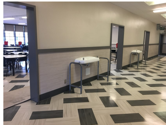
Completed finishes in Cafeteria
