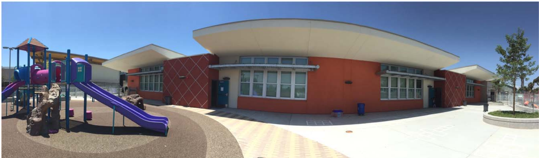
Panorama of building façade and playground
