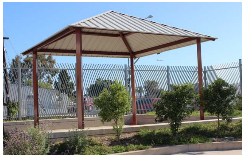
Shade structure on southwest side of campus
