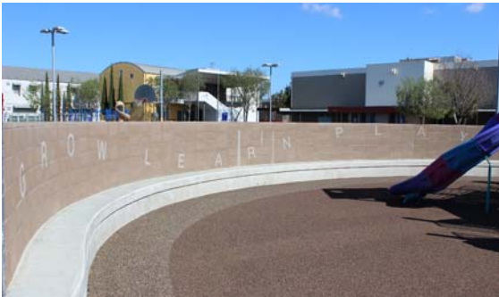
Custom boundary wall
