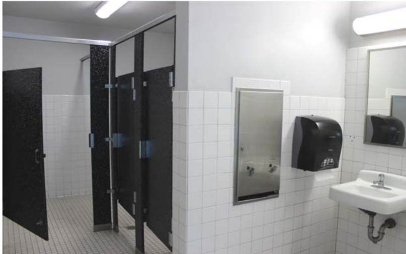
Remodeled girls bathroom
