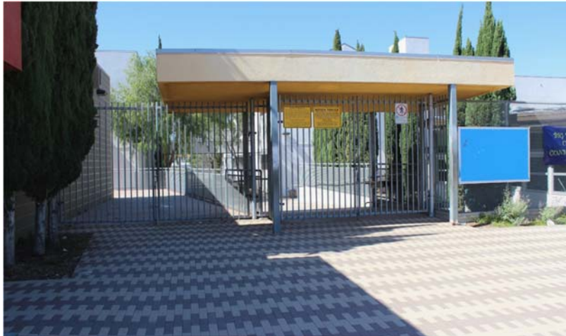
Front gate with upgraded security and custom pavers
