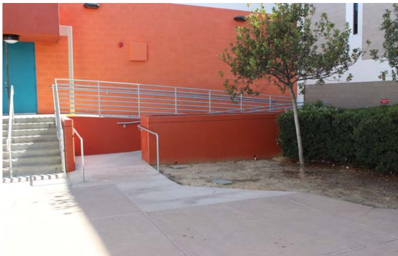
ADA ramp leading to administration building
