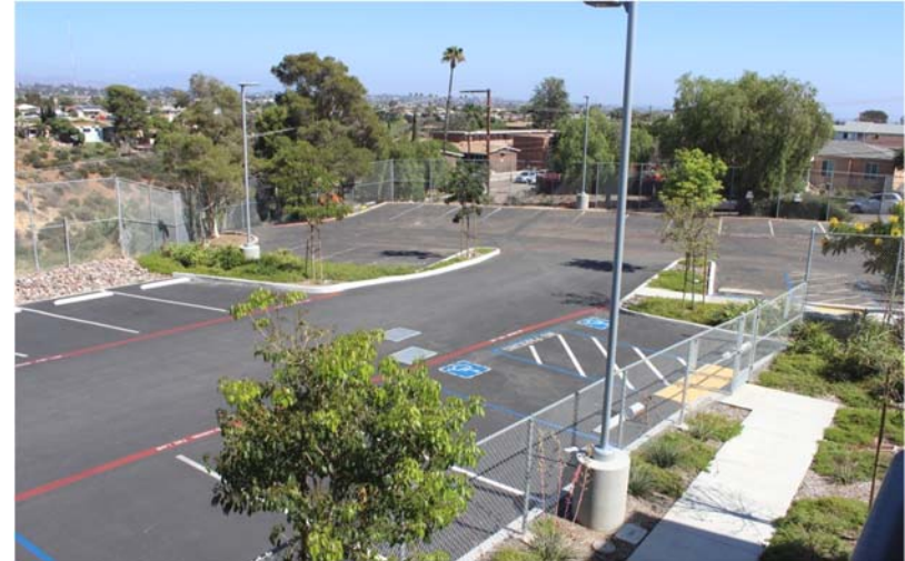
Expanded staff parking lot
