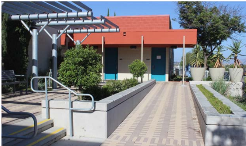
New entrance to office
