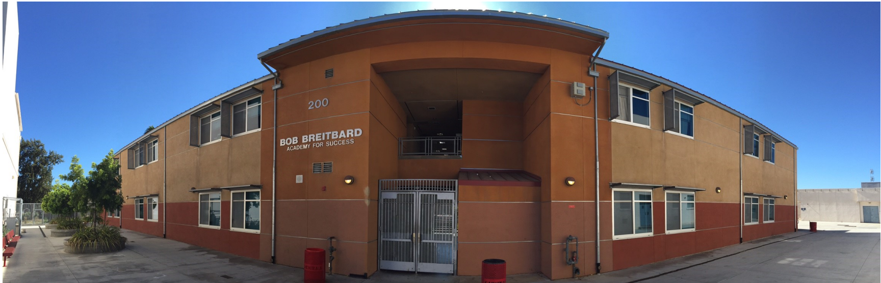
Panoramic of front facade
