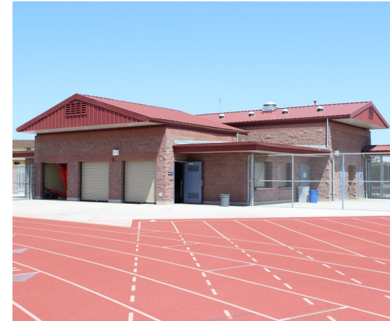
Athletic equipment storage
