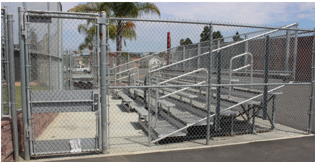
Bleachers with security fencing
