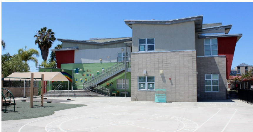
Staircase access to second floor
