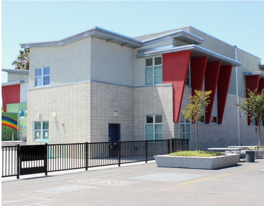
Building exterior (note the seam between the original and extension)
