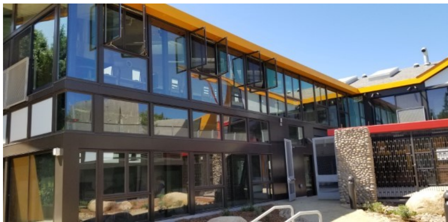
Main courtyard entrance
