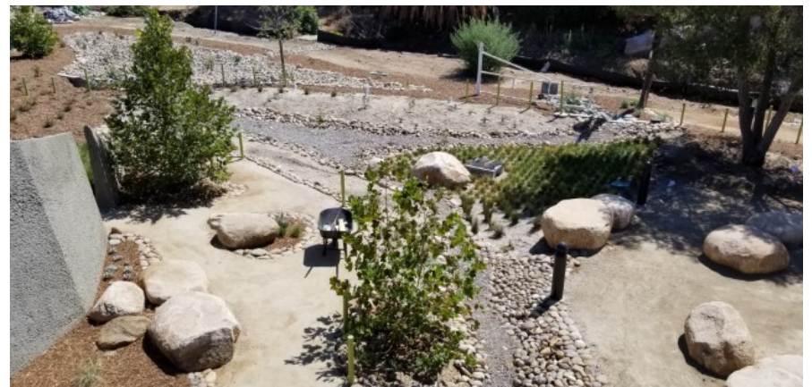
View of retention pond
