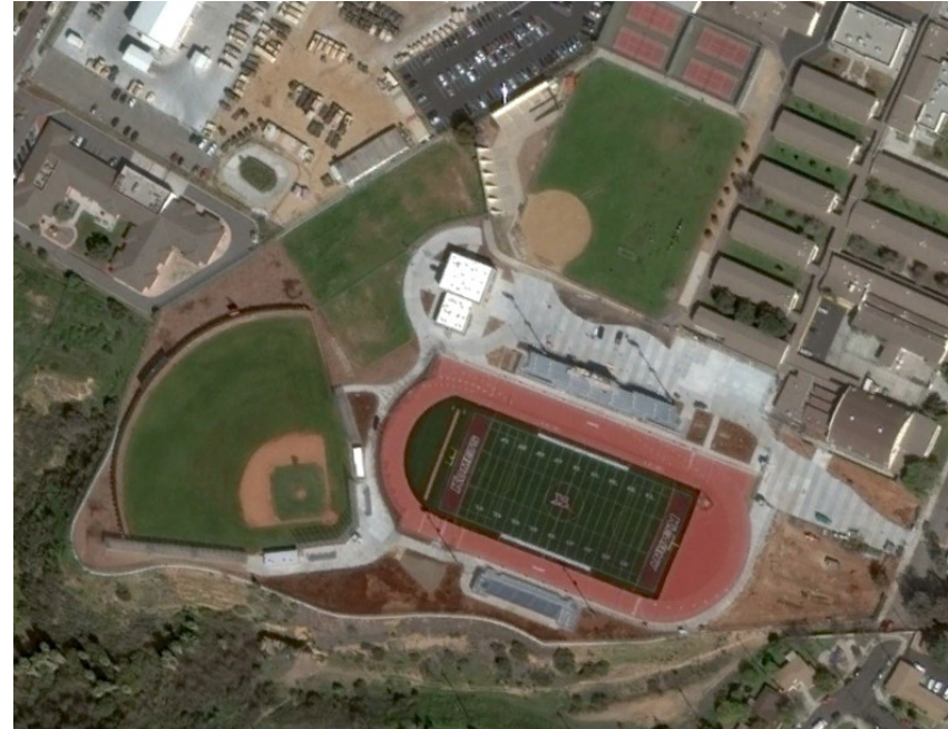
New fields and facilities, 2015
