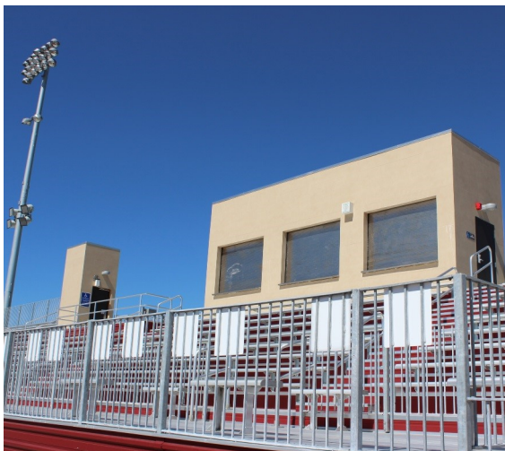
Press box and elevator
