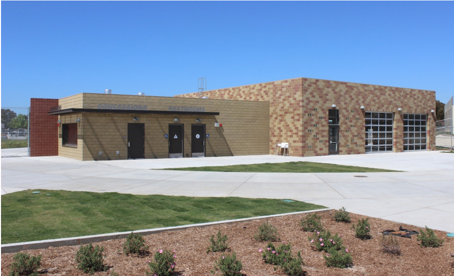
Concessions/restrooms and weight room facility
