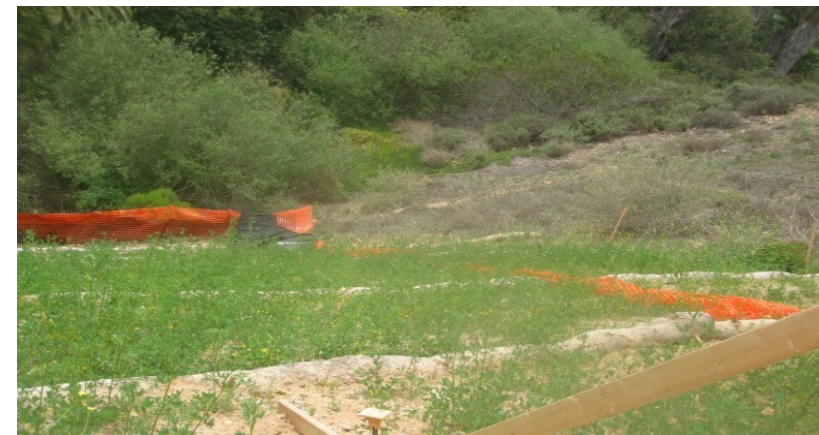
Hydro seeded plant growth
