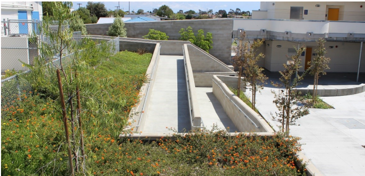
Example of ADA improvement
