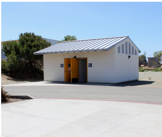
Restroom facility near field and lunch area
