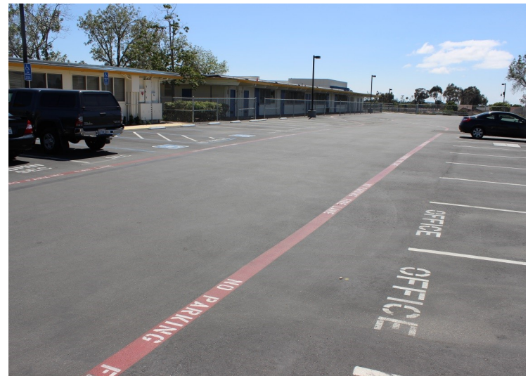
New parking with fire lane by administration office
