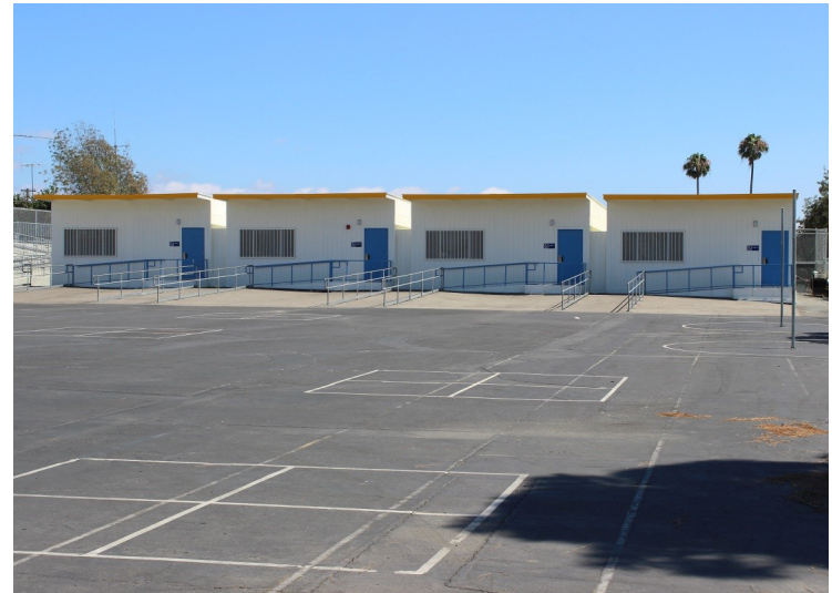
New modular classrooms
