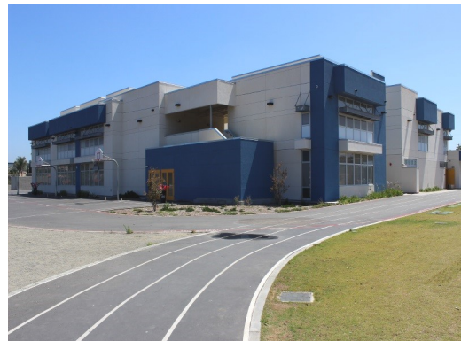
North and west side corner
