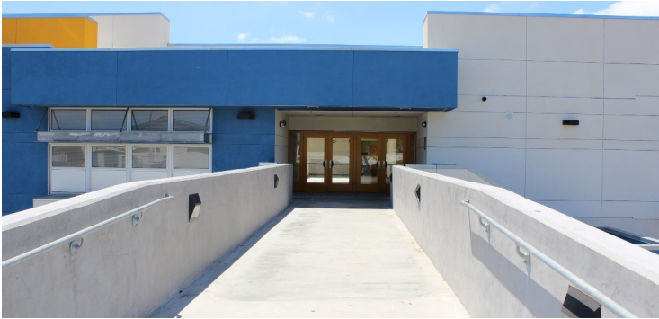
Second floor entrance
