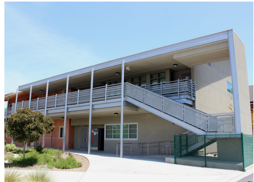
New 4,112-square-foot addition to 700 building
