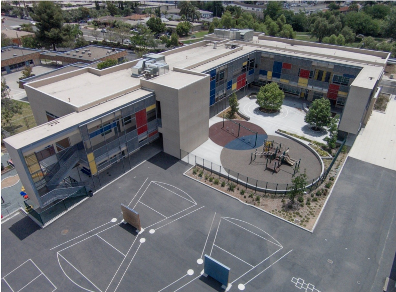
Aerial of new 24,761-square-foot classroom building
