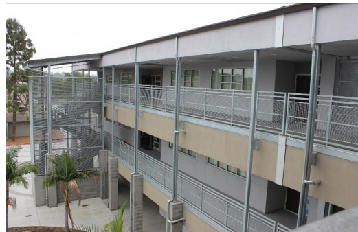
View of structure's three stories and staircase access
