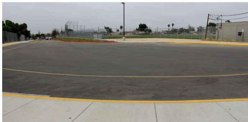
Turnaround with new striping and installed speedbumps
