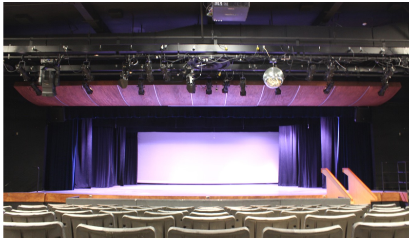
Theater with lighting and acoustic upgrades
