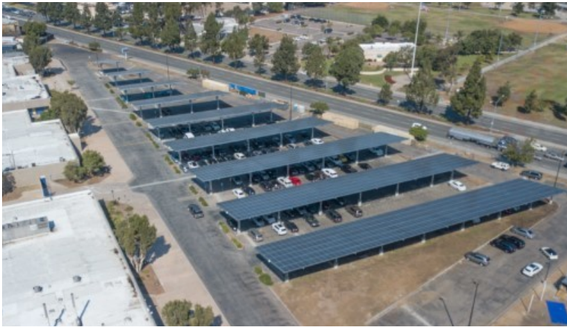
Solar Arrays on the Northeast parking lot
