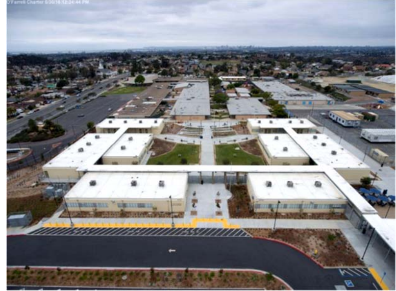
Aerial of new High School buildings looking west
