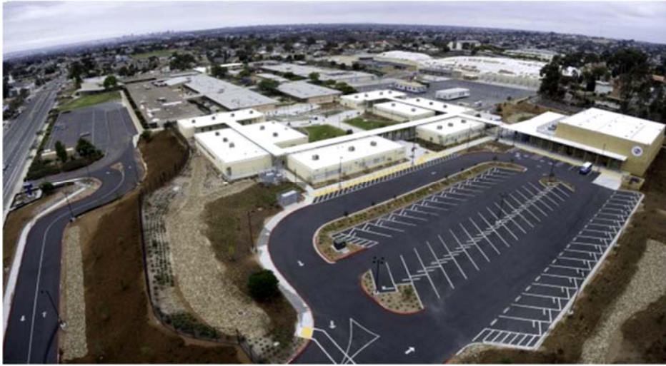
Aerial of new High School buildings, parking lot, roadway with new landscaping
