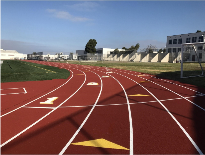
New track resurfacing and conversion to 400 meters
