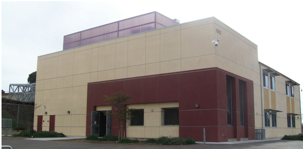
Completed building lower level
