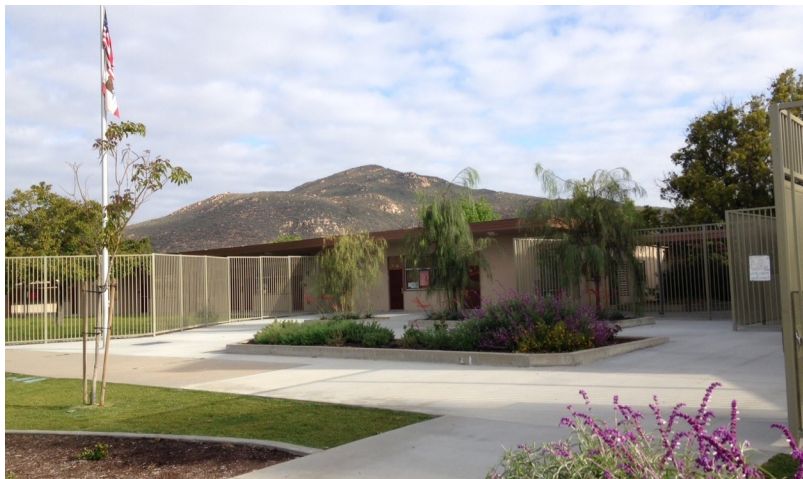
Front entrance security fencing
