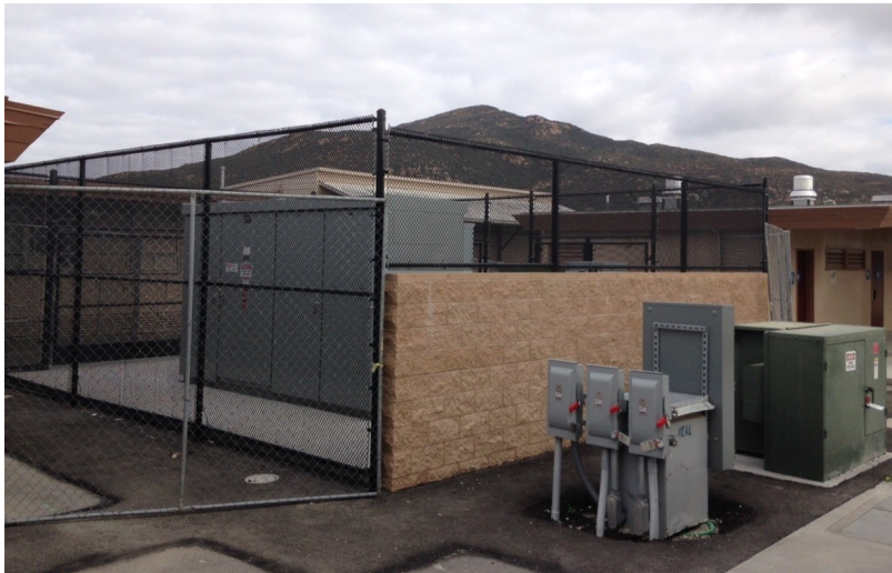
Electrical infrastructure improvements
