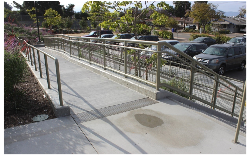
Front entrance Americans with Disabilities Act (ADA) ramp
