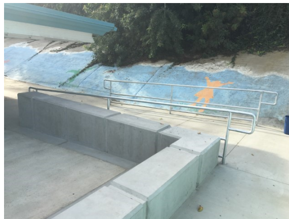
New concrete wall with ramp and railings
