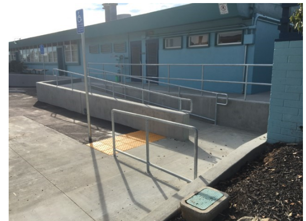
New accessible parking and ramp
