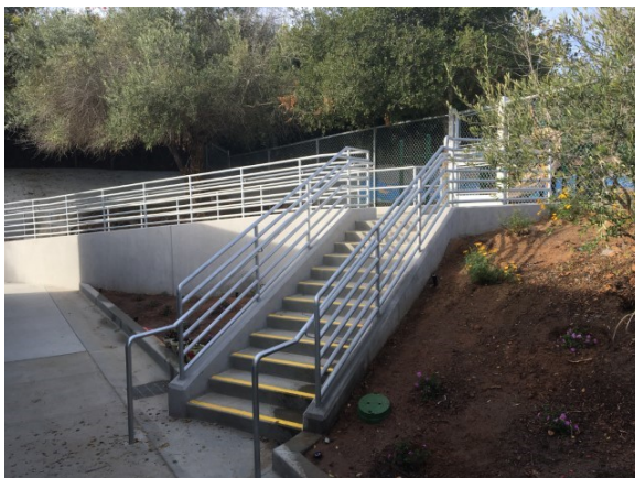
New stairs to Kindergarten building
