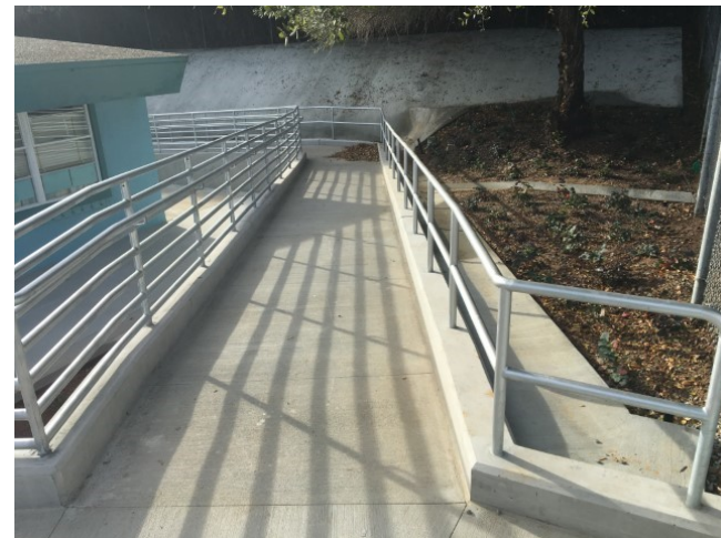
New kindergarten building ramp with landscaping
