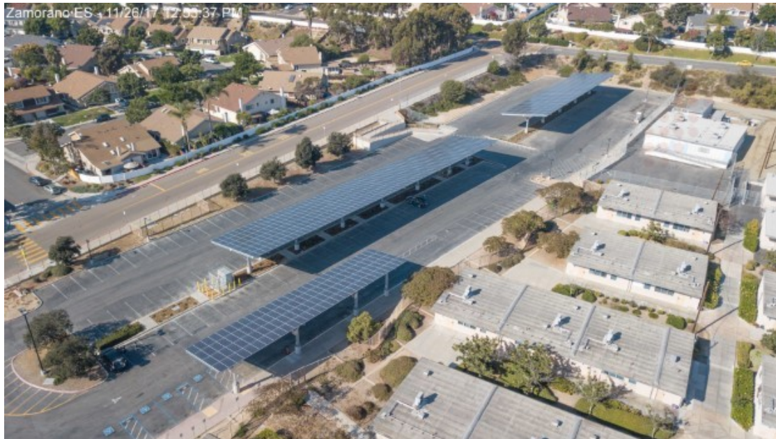
Solar Canopies on the Northwest parking lot
